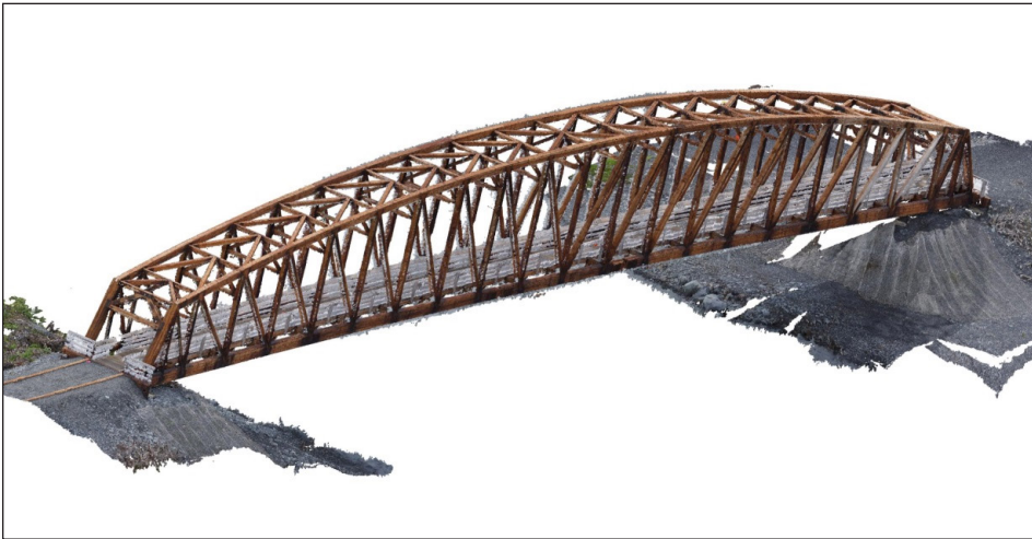
Figure 5 —A 3-D digital model of a bridge located just south of Anchorage, AK. PhotoScan was used to process both aerial and terrestrial imagery for a bridge inspection project. The imagery was taken using a Sony Nex7 camera mounted on a UAV and a handheld Nikon D800E camera.
